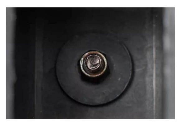
Inspect the nylon insert of the lock nut to ensure that it is intact after installation.
